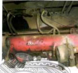
a. (5) (a) Broken Camshaft Support Bracket
