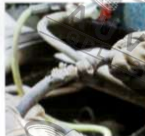
h. (4) Brake Hose Improperly Joined
